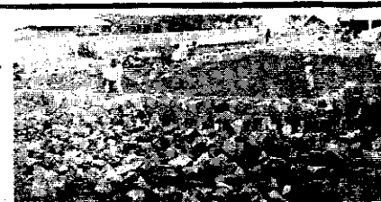
The foundation is prepared for the power plant from rocks that are plentiful around the village.
